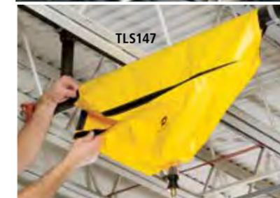
Standard funnel design (top) is made for single point leaks. TLS147 (left) wraps to catch spraying leaks.
